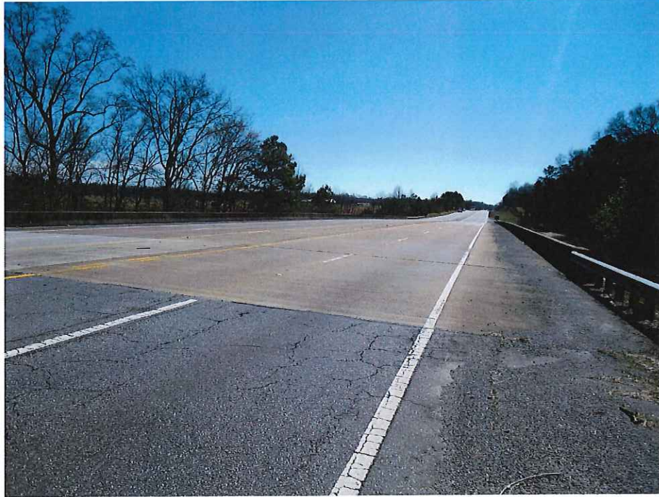
SR 1 (US 27) Looking East at Existing Bridge
