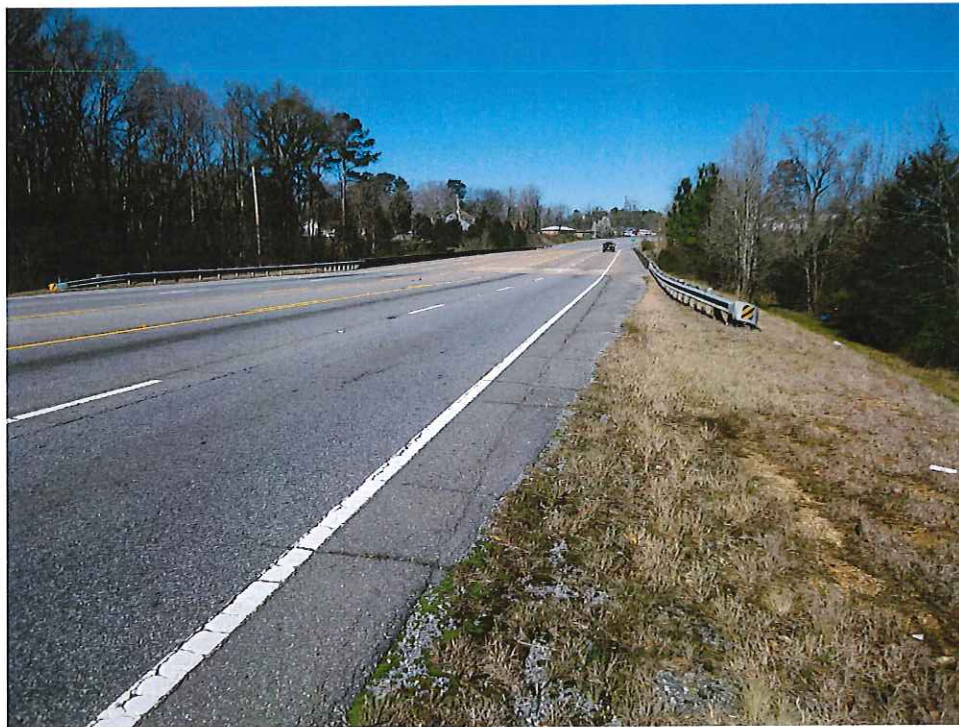
SR 1 (US 27) Looking West at Existing Bridge
