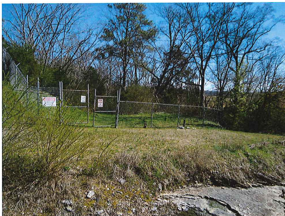
Downstream Floodplain West Side of Creek
