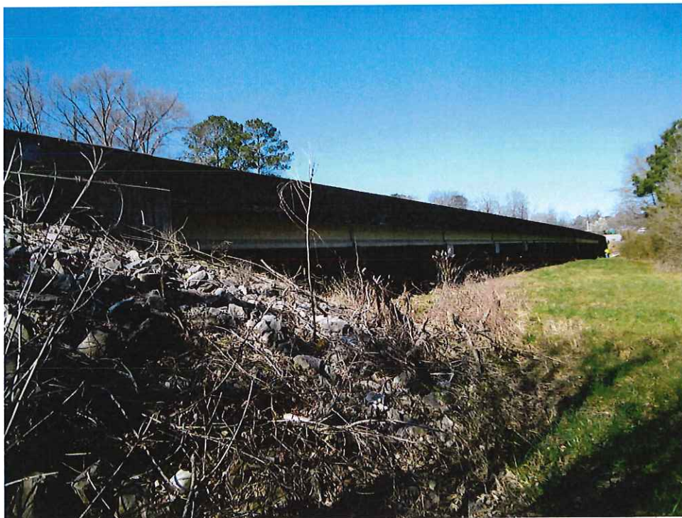
Downstream Face of Existing Bridge
